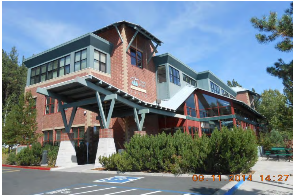
VIEW OF SUBJECT BUILDING LOOKING NORTHEASTERLY FROM NEAR DONNER PASS ROAD
