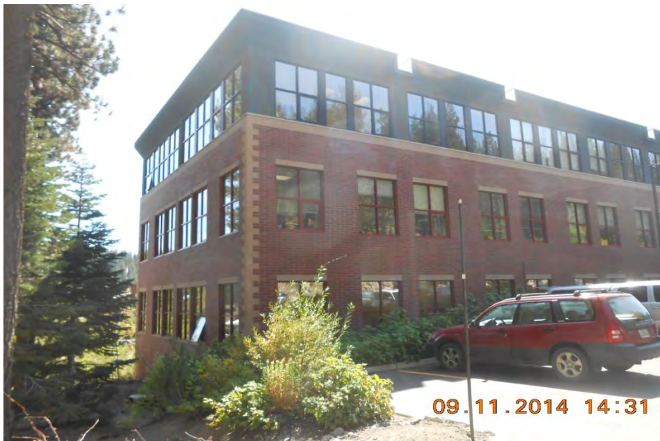
VIEW OF THE NORTHEAST CORNER OF THE SUBJECT BUILDING, SHOWING THE SUBJECT SUITE ON THE 3 RD FLOOR, LOOKING SOUTHWESTERLY FROM THE EASTERLY PORTION OF THE PROPERTY
